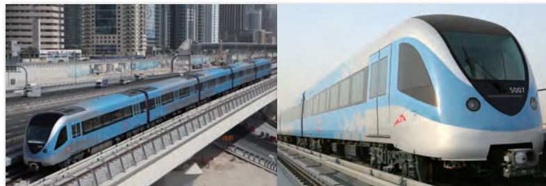
• Dubai Metro (fully automatic unmanned operation, EPC full turnkey project, completion with delivery ahead of schedule)
